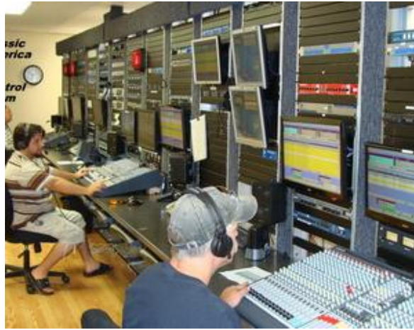
TOC, Technical Operations Center
